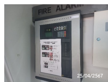
Fire Alarm Control Panel
