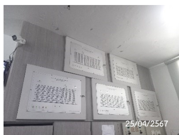
Graphic Annunciator Fire Alarm
